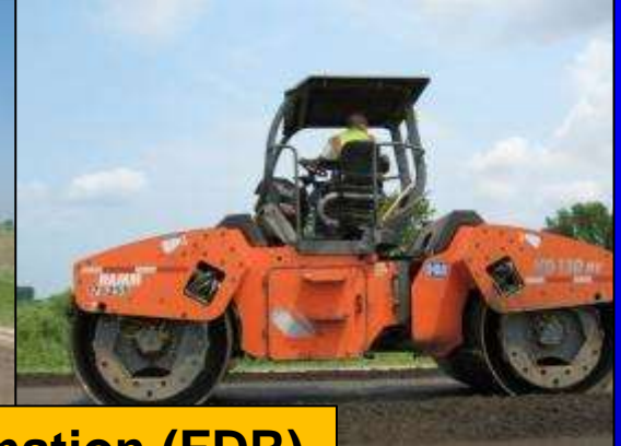
Stabilized / Un-stabilized Full Depth Reclamation (FDR)
