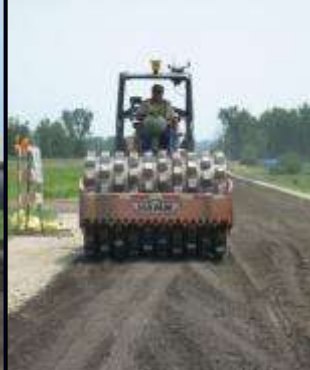
Stabilized / Un-stabilized Full Depth Reclamation (FDR)
