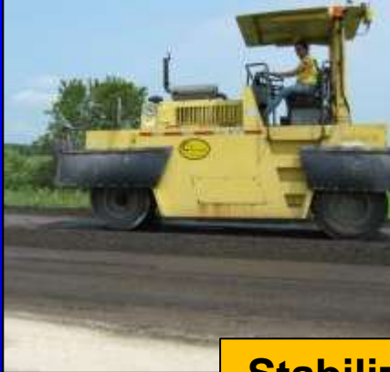
Stabilized / Un-stabilized Full Depth Reclamation (FDR)
