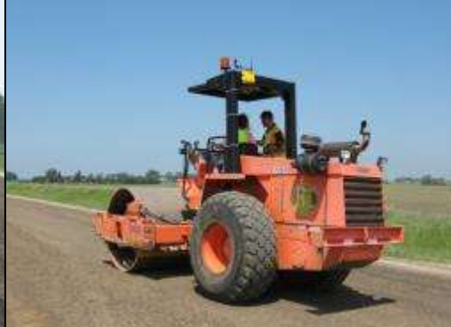
Stabilized / Un-stabilized Full Depth Reclamation (FDR)
